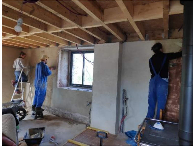
A 3SR worksite.
